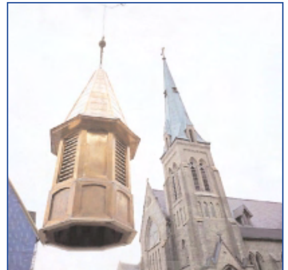
Photo: Philip Lengden Raising the cupola on the New Residence
