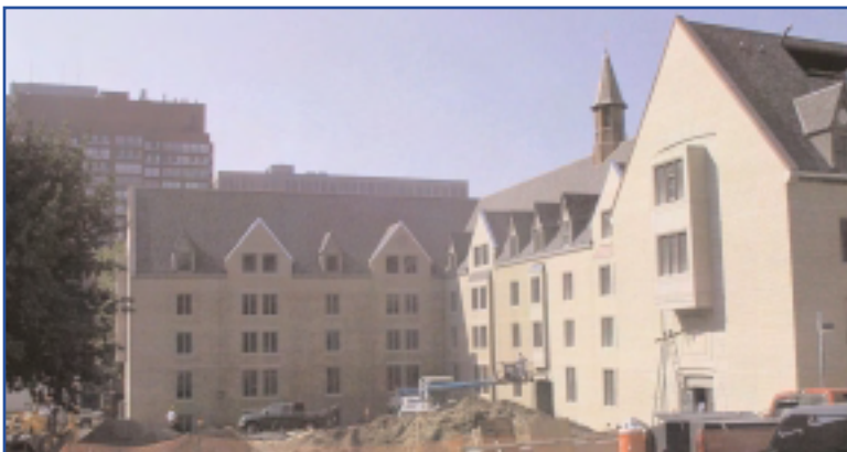
New residence from the east
