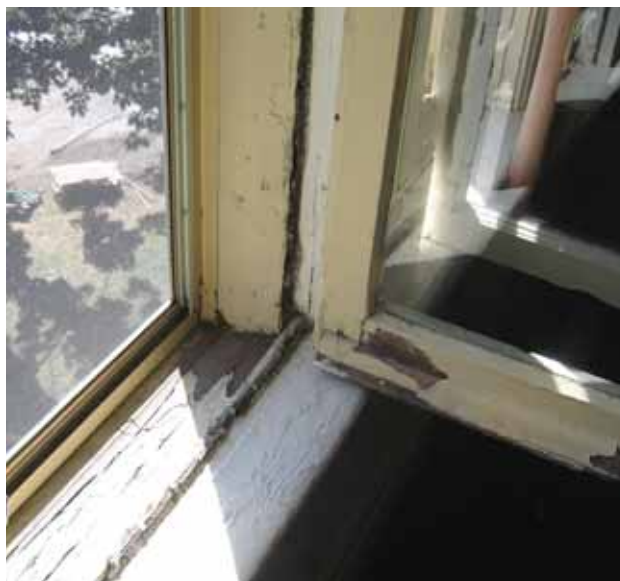
Showing signs of wear and years of water damage
